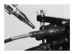
11.12 Wait until the sleeve is cool to the touch before moving the cables.
